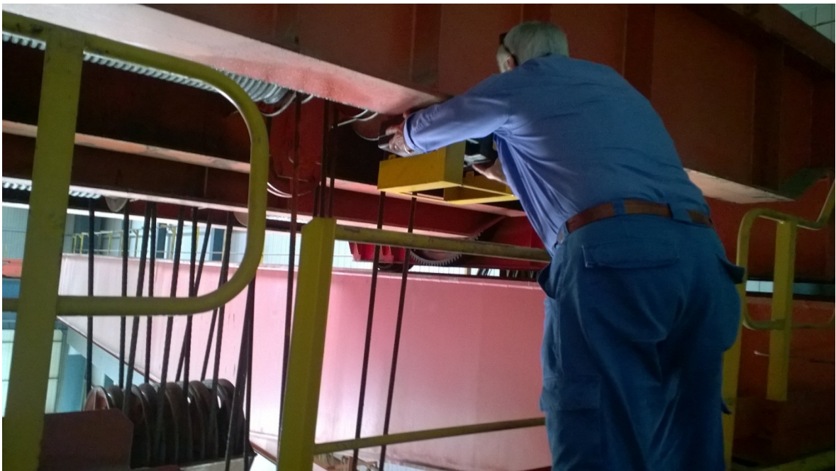
Figure 22. Installation of the prototype by the crane-operator.
