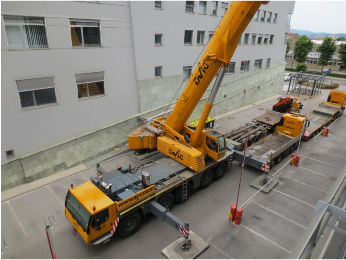
Figure 4. Operating crane Liebherr LTM 1200-5.1.
