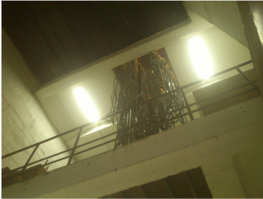
Figure 14. The lowest level of machine hall served by the selected crane (view from lower level).
