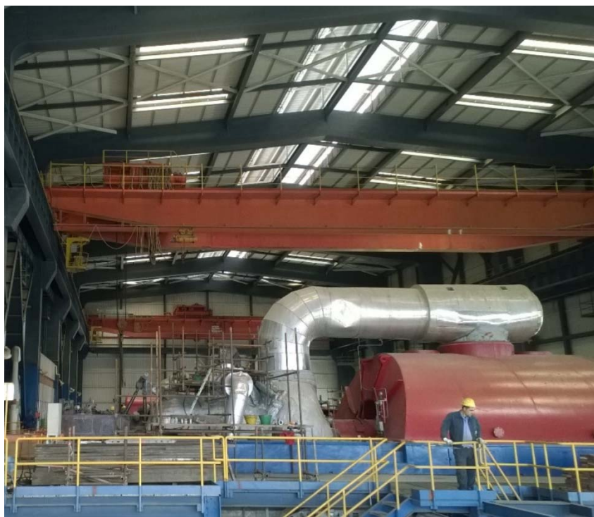
Figure 6. Selected crane in the Edipower Company (Galileo 150 60 51).
